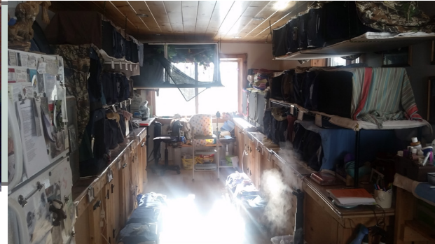
Finding a home: A dilapidated, poorly constructed room with a leaking roof was transformed into the hospital room in 2009. Last winter it was a hibernacula for 96 bat patients with temperature maintained between 45-50° Fahrenheit, and kept at 60-80 percent humidity, to try to mimic a cave setting.
